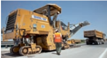
KM 142 A PM200 paver at work
