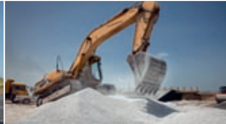
KM 152 A hydraulic excavator moves stone into position ready for spreading.
