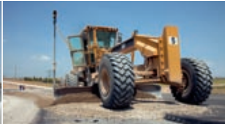
KM 150 Levelling in progress with a 16H motor grader.
